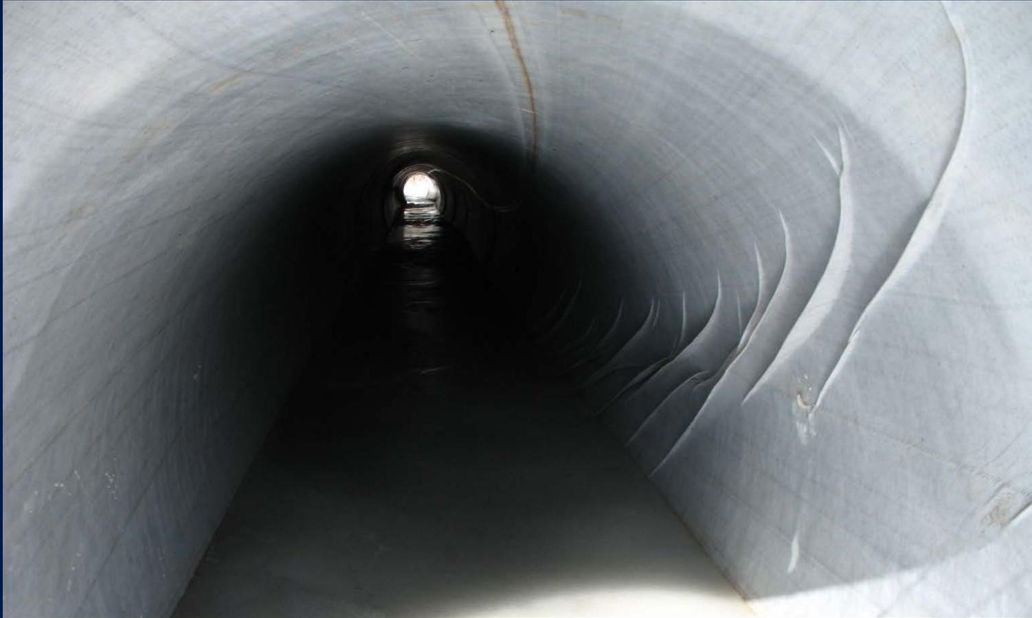
CIPP Liner is resin-filled fabric, inflated and cured with hot water or steam or UV light till it's rigid
